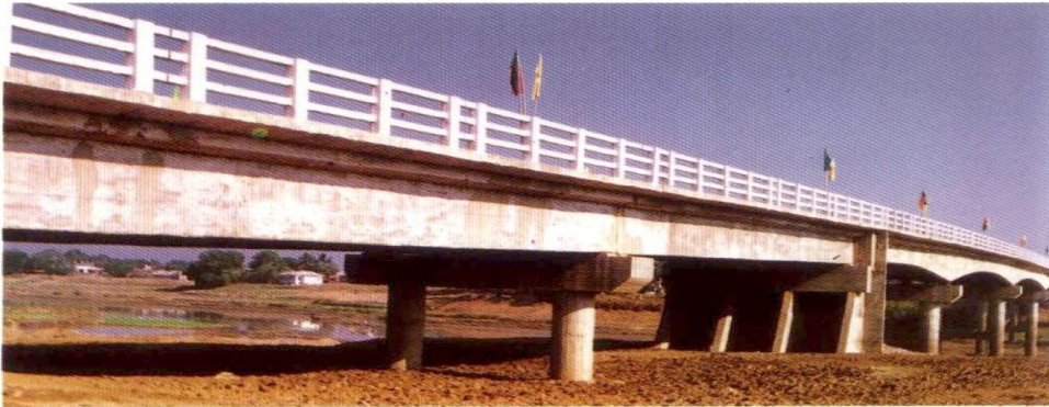
Pre-Stress Girder Bridge on Dhaka Mymensingh Road
